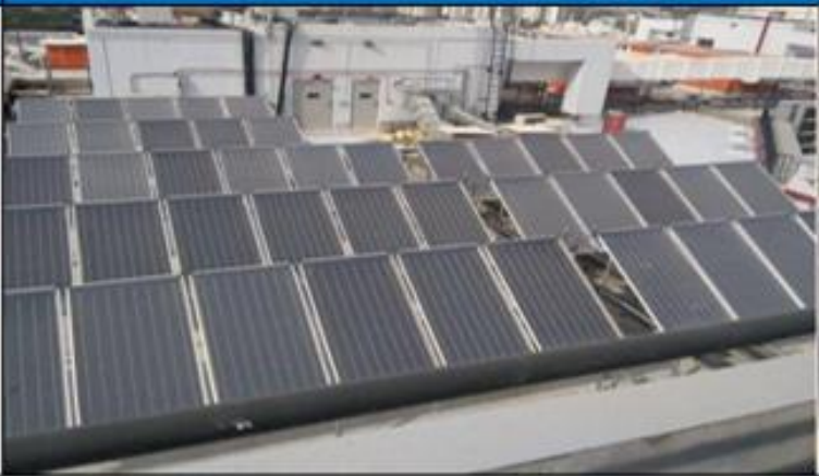
SOLAR THERMAL supplies 100% domestic hot water supply
